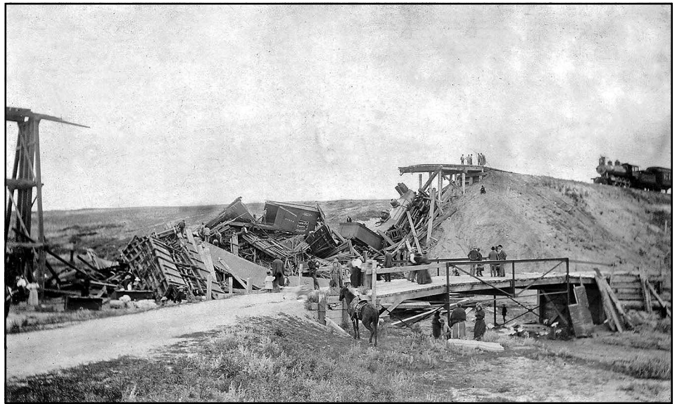
The great Santa Fe train wreck of July 17, 1895 occurred about 1/4 mile south of today's 2nd Street / Beacon Lite Road north of Colorado Springs. —Photo Courtesy of The Vaile Museum
